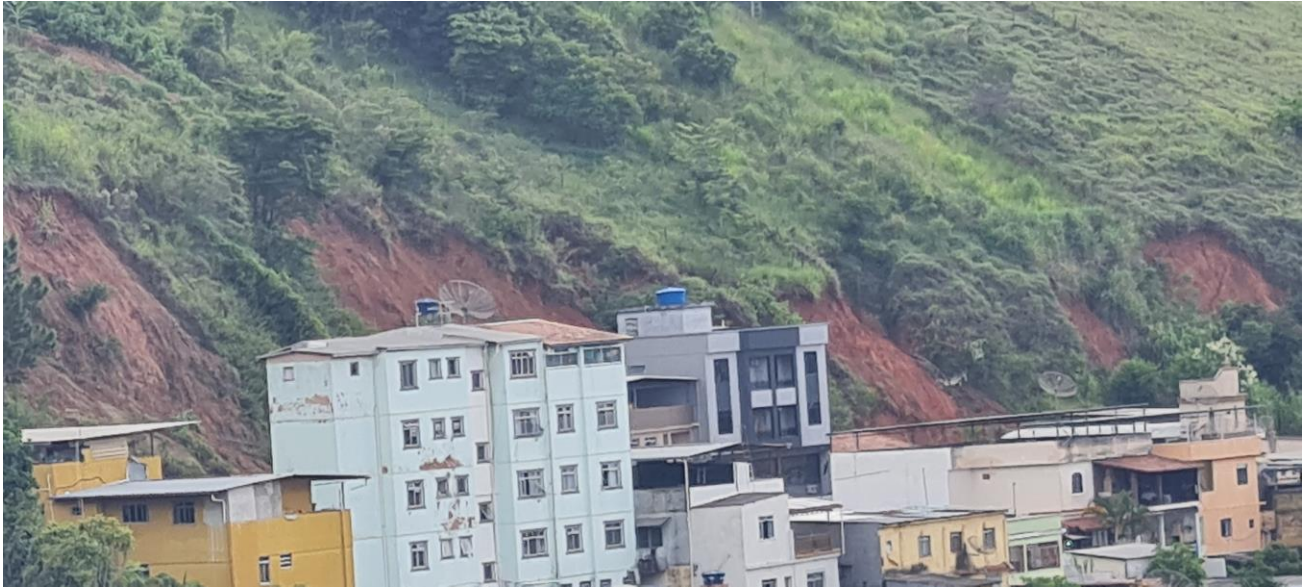
Figure 1 – Landslides affecting the urban area of the city of Juiz de Fora during CENACID's emergency mission in response to the disaster that struck the state of Minas Gerais. CENACID provided scientific support to the municipality during this major disaster in February 2026.
