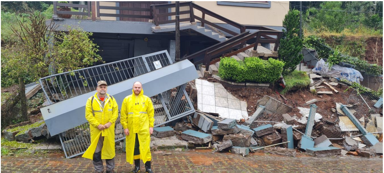
Figure 2 - House destroyed by a landslide during the catastrophic event that hit the Rio Grande do Sul State in May 2024.
