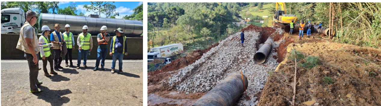
Figure 1 - Field research in cooperation with road system engineers and geologists (left). Providing scientific support to the State of Rio Grande do Sul during the major disaster of May 2024, when a landslide destroyed the water supply system (right).
