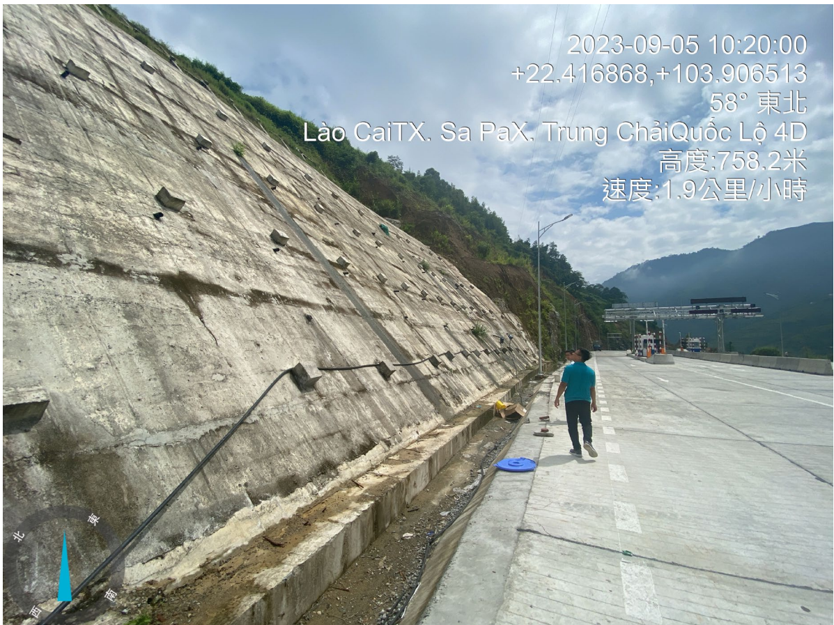
Mong Sen Roadside slope failure and retaining wall construction
