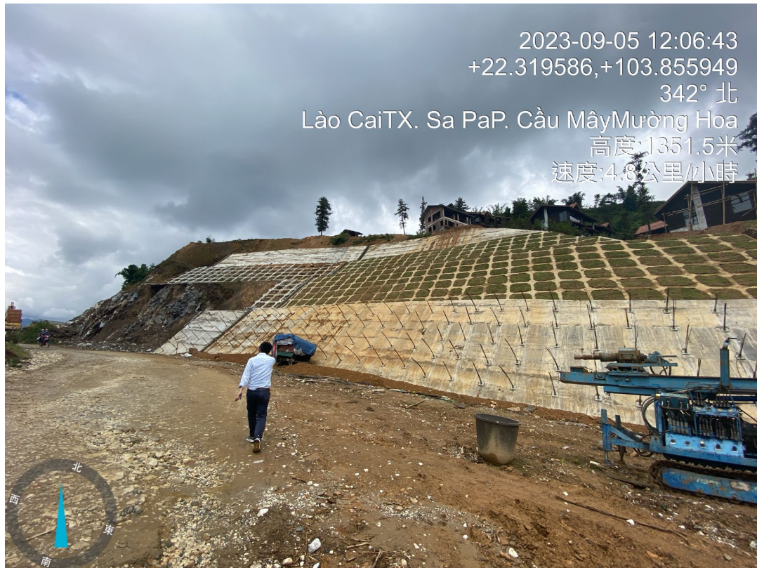
Caumay ward Construction of roadside retaining wall
