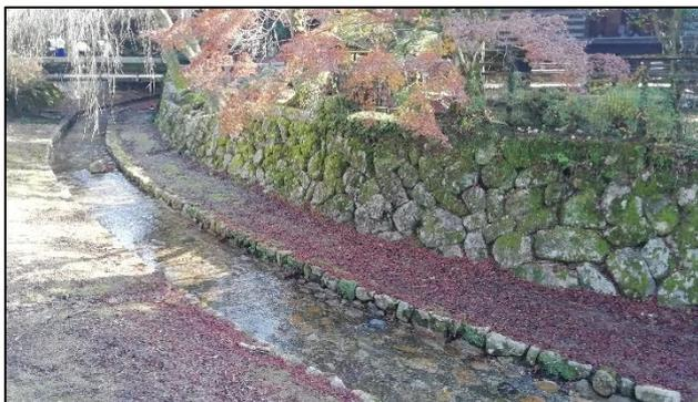
*Image 2 – Application of erosion control measures to the river bank and bed of Momijidani River.*
