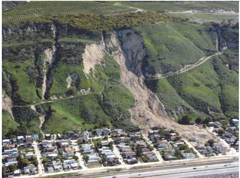
Figure 1. This landslide occurred at La Conchita, California, USA, in 2005. Ten people were killed. (Photograph by Mark Reid, U.S. Geological Survey.)
