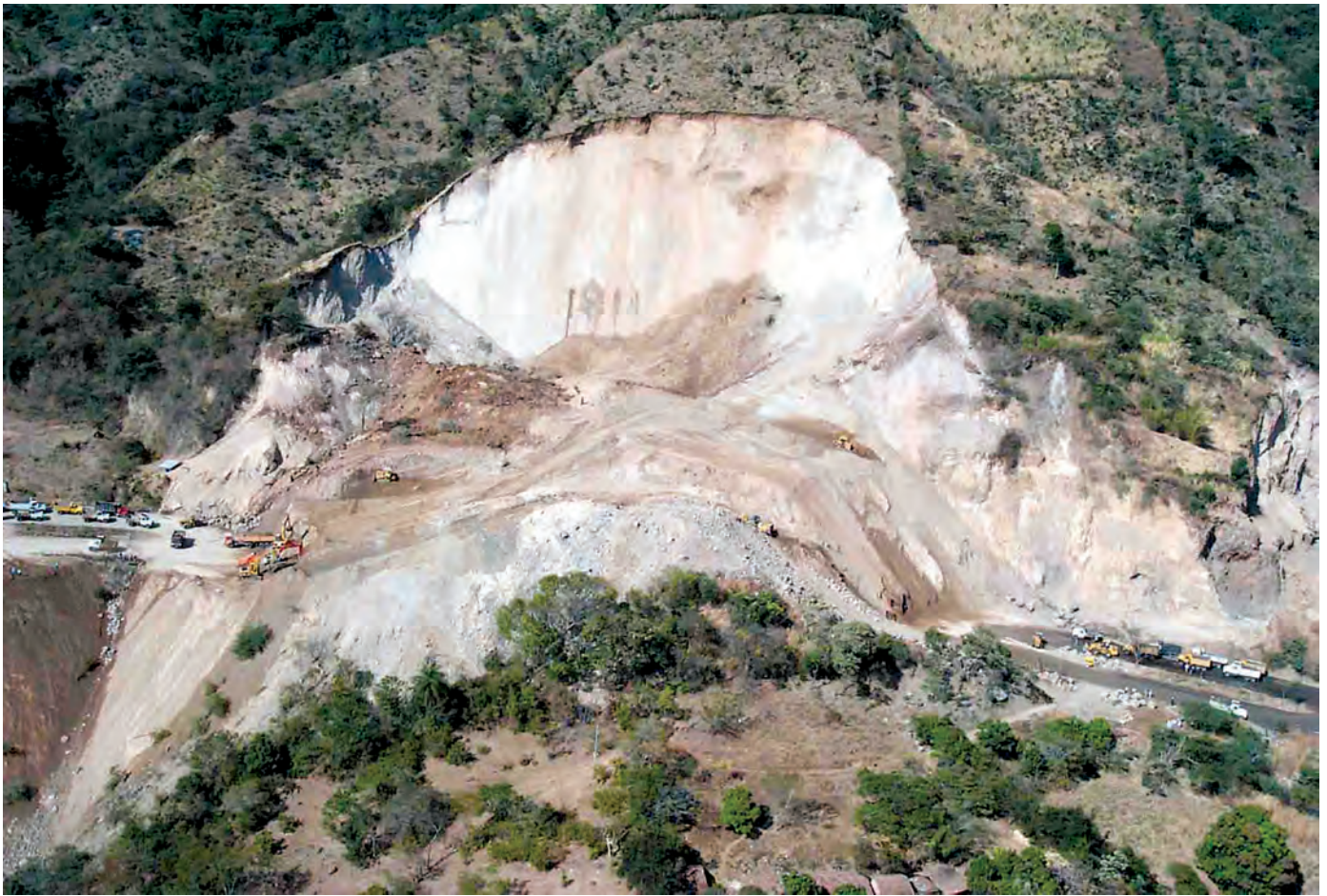
Figure 29. A landslide on the Pan American Highway in El Salvador, Central America, near the town of San Vicente, in 2001. (Photograph by Ed Harp, U.S. Geological Survey.)
